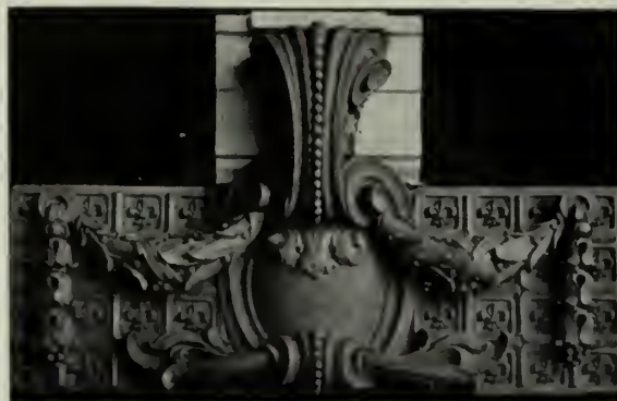
DETAIL BY WHEELER, GALLEHER & STERN, ARCHITECTS. New Jersey Terra Cotta Company, Makers.
